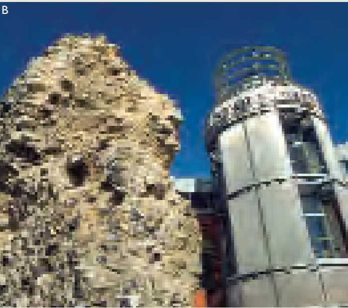
B The Chapelfield development, situated within the context of the city wall
