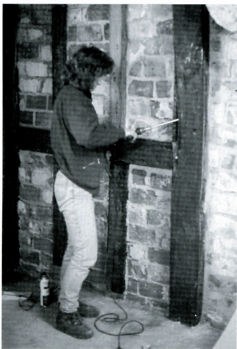
Dendrochronology: taking samples from in-situ timber framing, Walmgate Bar, York
