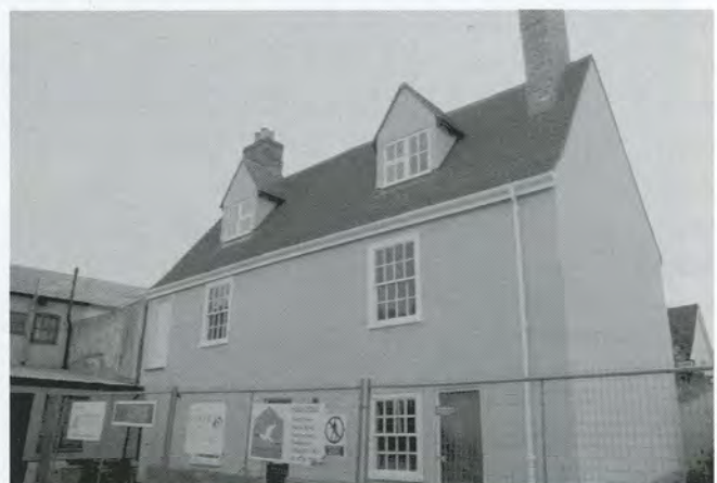
Working closely with the Housing Department brings results - Bury-St-Edmunds
