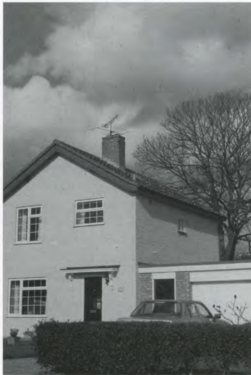
Look at the effectiveness of the boundary - this house has been built right on top of it (Horringer)
