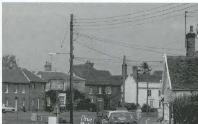
Select suitable locations for under-grounding cables - Cavendish
