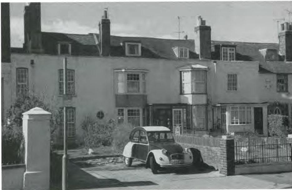
The removal of boundary walls and the use of front gardens for car parking can be visually intrusive and can be controlled by the use of Article 4 Directions (Deal)
