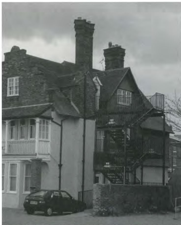
The provision of most fire escapes will have a material effect on the appearance of the building and will require planning permission (Deal)
