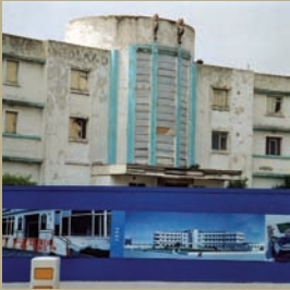
Midland Hotel, Morecambe - re-use of existing buildings can be more sustainable than new build, whilst retaining local identity
