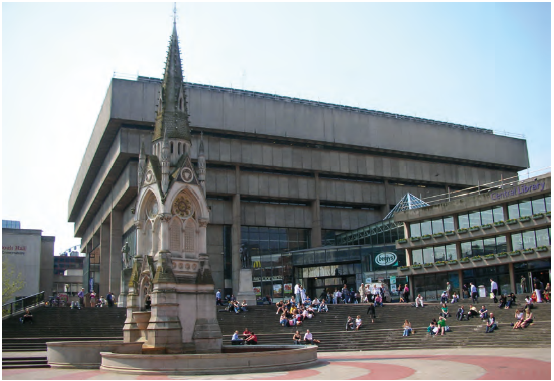
Figure 6: Central Library, Birmingham, by John Madin, c. 1973. Hoardings going up for demolition in March 2015 (photograph: author).
