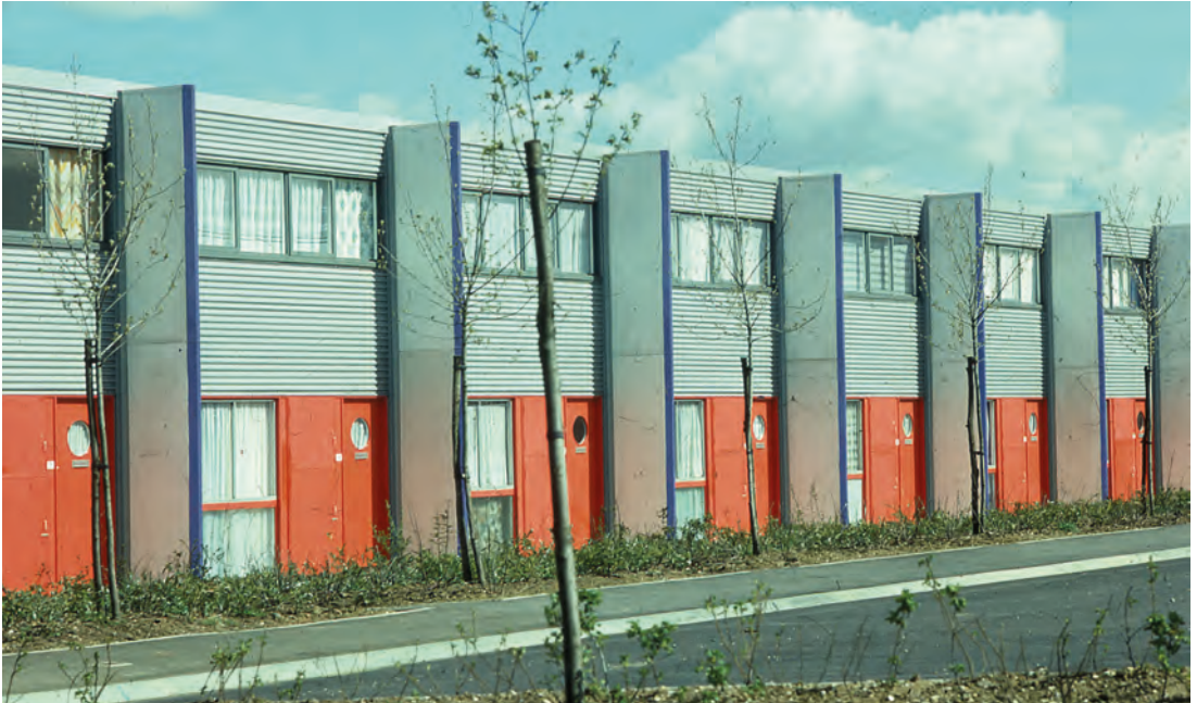
Figure 5: Netherfield houses, each dwelling divided by a fin with primary colour highlights, as photographed by John Donat in 1973. Image courtesy of Milton Keynes City Discovery Centre under Government Open Licence v3.0 (MKCDC Ref: Ca-4991)
