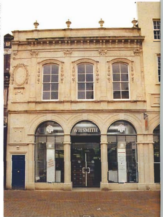
New shopfront restores the architectural relationship between ground and upper floor
