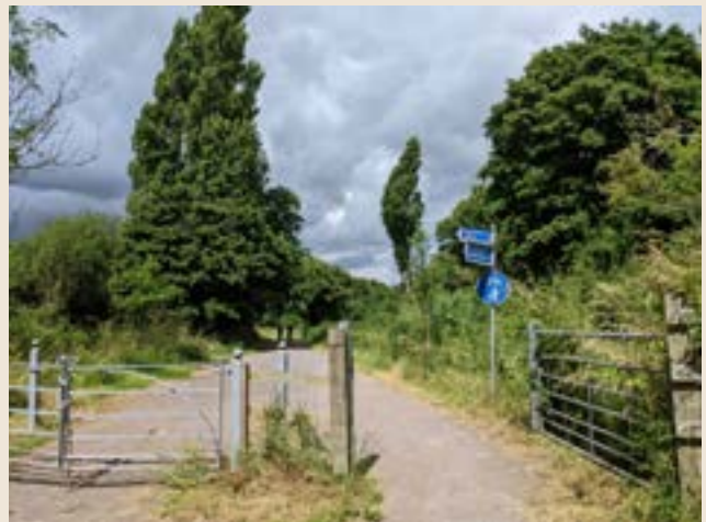
Figure 67 Re-using former railway corridors as cycle paths, funded by new housing development in Wells
