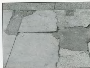
31. (bottom) Attractive steps replaced with concrete and quarry tiles.
