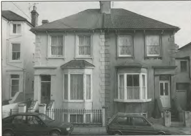
15. Houses in Hove badly affected by replacement windows, painting, concrete roof tiles and the removal of railings.
