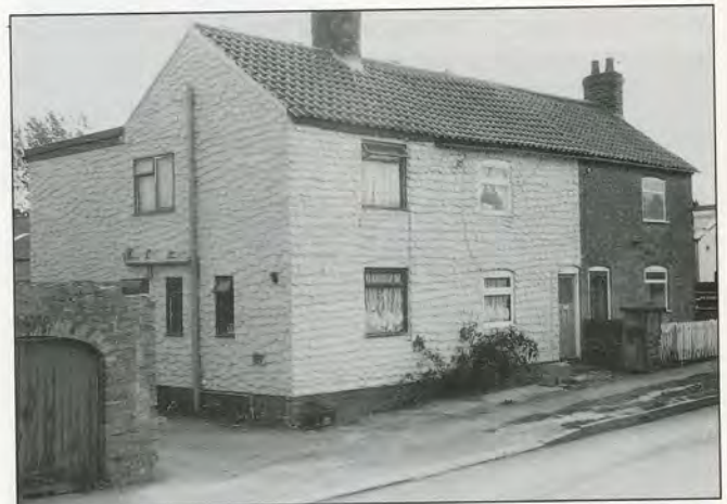
14. (right) Thick render, replacement windows and missing garden fence ruin the appearance of this house in Beverley.
