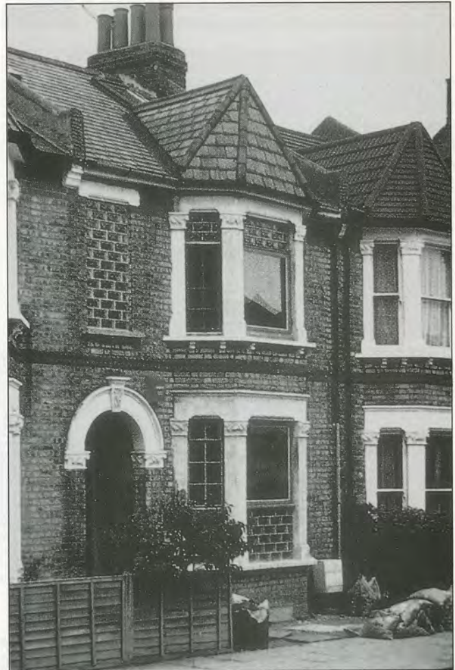
16. 'Traditional Homes' magazine has a feature entitled "Mess of the Month". A reader sent in this picture of a property in West Hampstead. The alterations using glass bricks would be permitted on an unlisted house in a conservation area.
