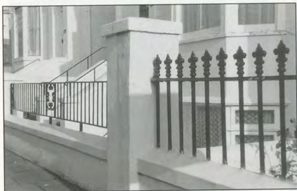
25. (above) Victorian cast iron railings removed.
